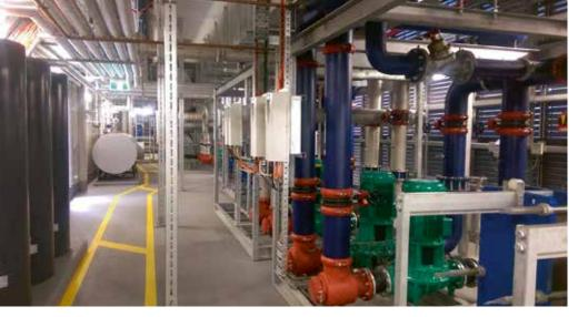
The use of pre-fabricated pump skids helped minimise the on-site installation times at 180 Brisbane. Image: A. Gatland, AE Smith.
